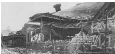
Franklin Marshall School (After)
